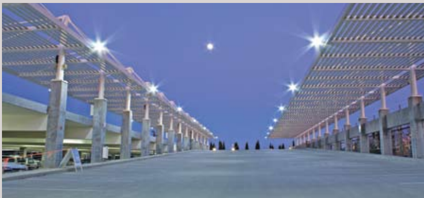
The lighting in the parking structures at UC Davis provided an opportunity to implement cutting edge technology.
